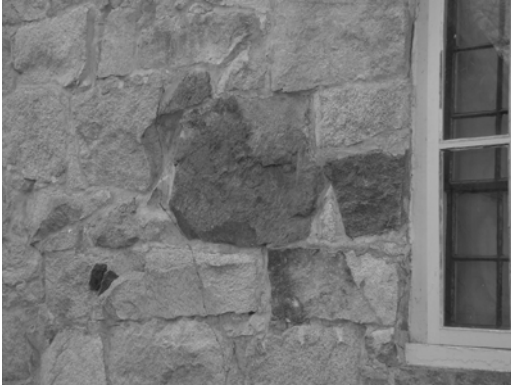
Figure 5 - The church's north wall shows a great variety local stone, of different "shapes." Also note the absence of drill marks.
