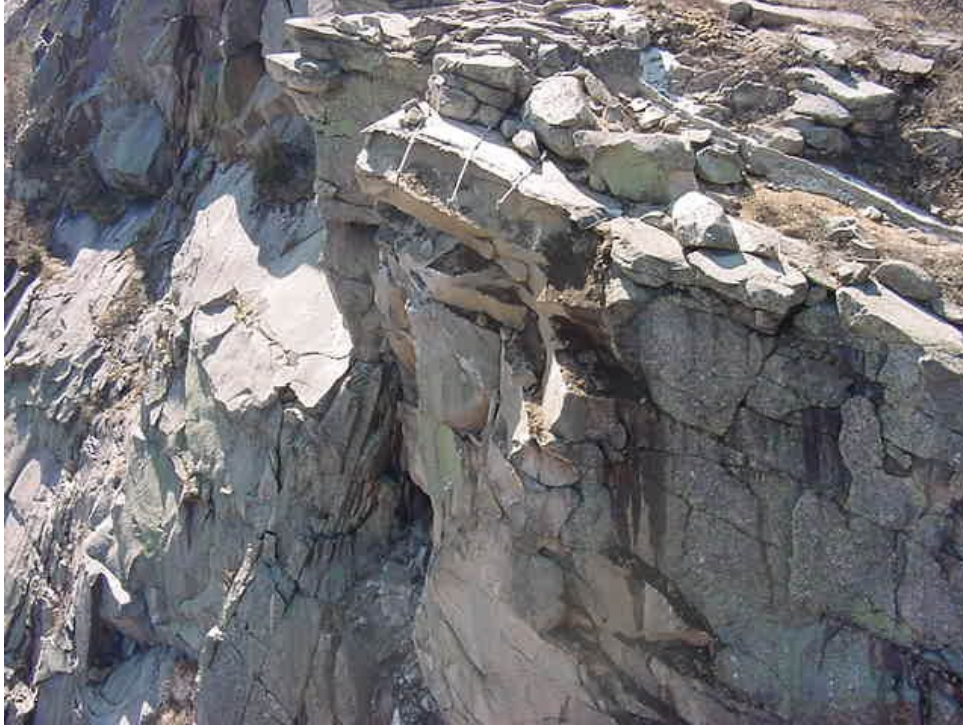
Fig. 2. All that remains of the Old Man after May 2-3, 2003. Note the three remaining steel rods that had been installed to hold the rocks of his forehead from sliding. (Photograph courtesy of George Bliss.)
