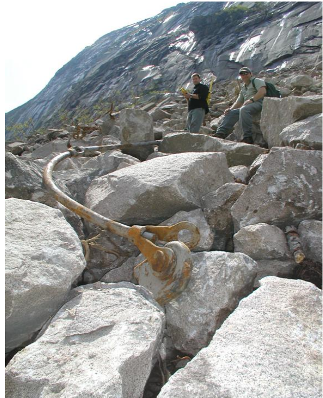
Fig. 2. All that remains of the Old Man after May 2-3, 2003. Note the three remaining steel rods that had been installed to hold the rocks of his forehead from sliding. (Photograph courtesy of George Bliss.)
