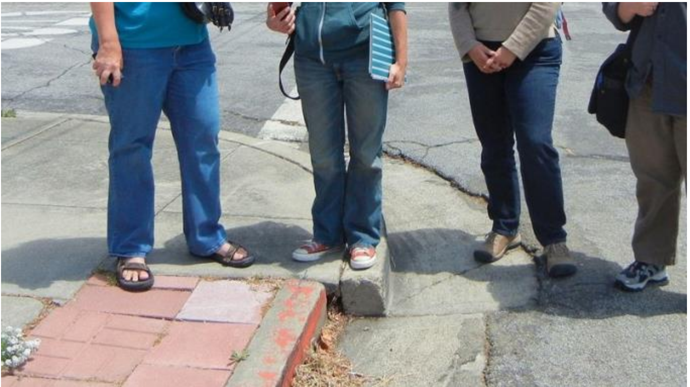
Geology enthusiasts gather at a (formerly) noteworthy curb in Hayward, Calif., in May 2012. The curb was once straight; the shifting Hayward fault pulled it apart
