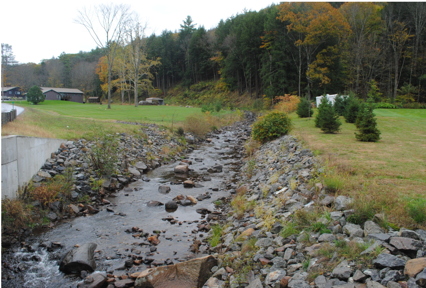
TRIP A-1 - Warren Brook, Alstead, NH impacts and recovery efforts after the 2005 flooding, Sean Sweeny and Lindley Hanson leading. Photograph shows a segment of Warren Brook that was stabilized with riprap immediately after flooding. Contrast these conditions with those shown in the next photograph.
