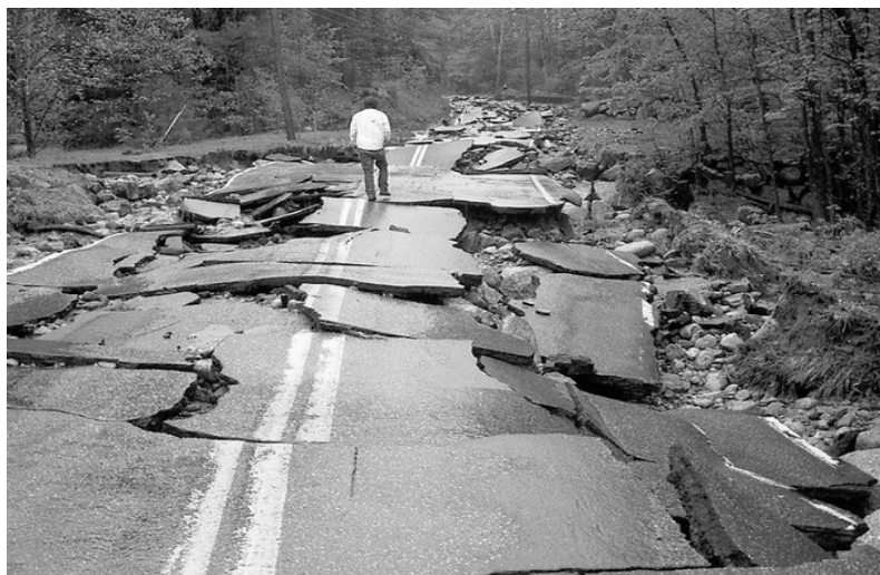
Photo 4 - A Road in Henniker, New Hampshire after the May 14, 2006 Mother's Day Flood ( Source: Accuweather ).
