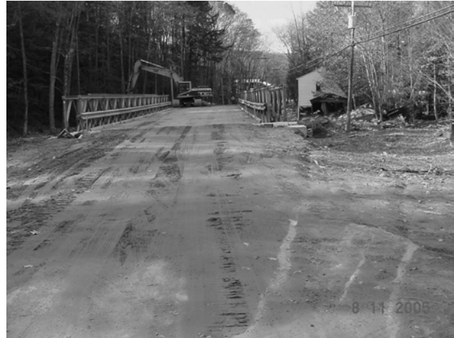
Photo #6B (Right) Temporary Bailey Bridge installed at Warren Brook culvert pipe crossing. (Photo by Dick Lane – NHDOT.)
