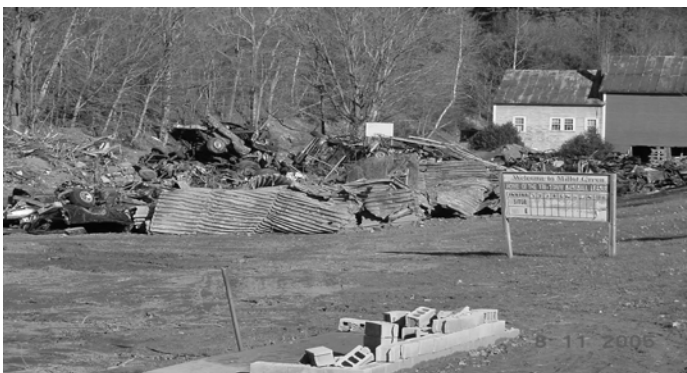
Photo #4. Piles of scrap metal and cars at Alstead parade field. (Photo by Dick Lane – NHDOT.)
