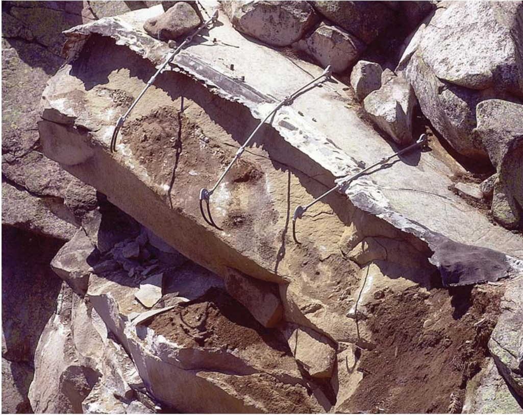
Figure 9. Close-up, top of the Profile's residual rock mass (photo by Union Leader Corp., 2003).
