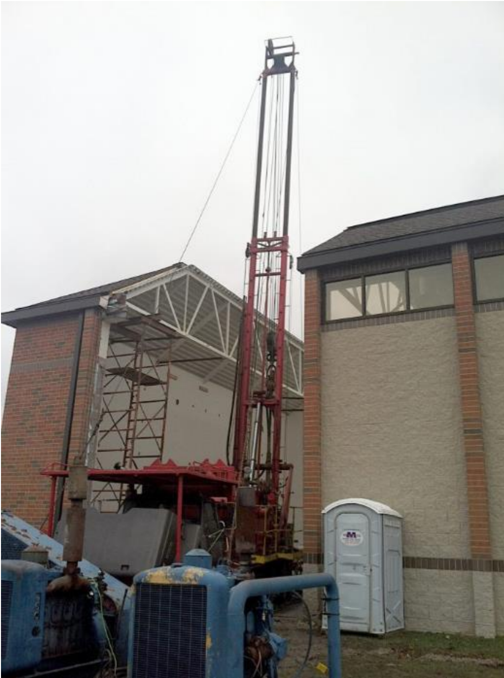
Workers plug a natural gas well at an elementary school in Lorain, Ohio in 2015. The recently constructed school had to be evacuated when the well, located underneath the gym floor, began leaking gas. Credit: Ohio Department of Natural Resources
